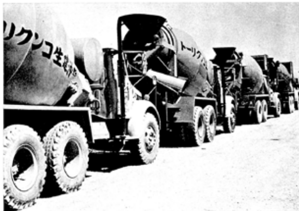
Model HF concrete mixer trucks lined up for work on the island of Okinawa where a large-scale construction project is underway.
