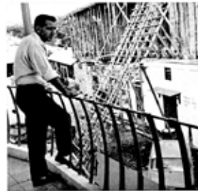
John Michael, president of Michael's Stores, watches construction work in progress on his new company headquarters building in the city of Bo, Sierra Leone, West Africa. Michael will deliver new HINO Motors large-size buses and trucks to customers engaged in building and developing the new nation.
